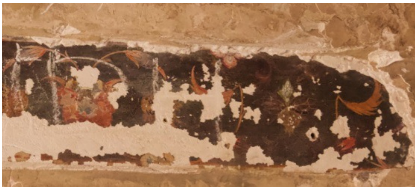
Figure 10 Western chamber. Painted panel. Flaky painted layer hidden behind thick plaster. Detailed floral study.
