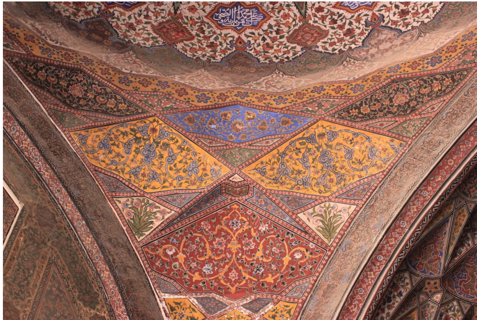
Figure 17 Wazir Khan Mosque Ceiling
